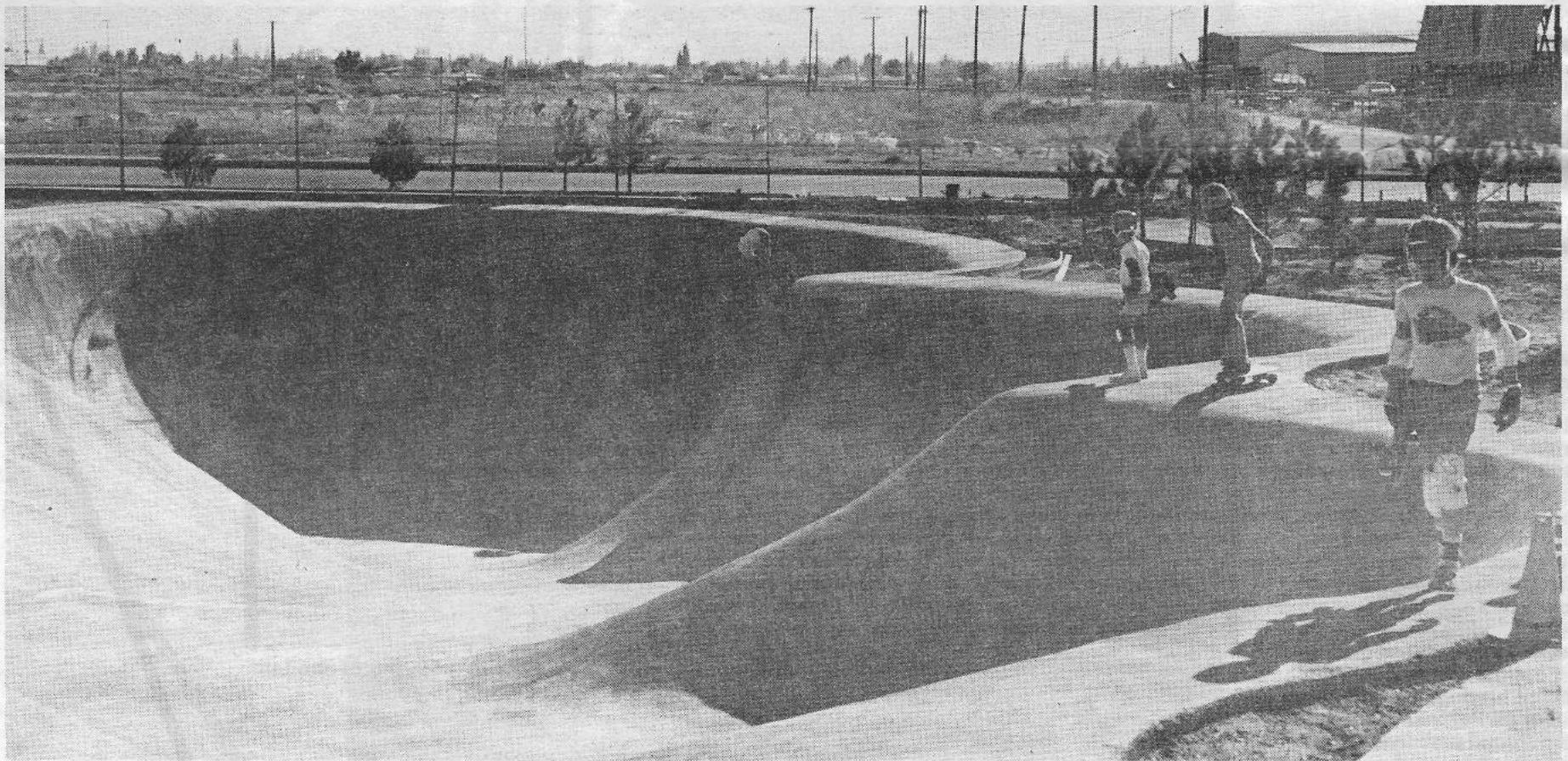
Surface shot of one of the bowls at Blue Skies Skatepark, Albuquerque, New Mexico.
